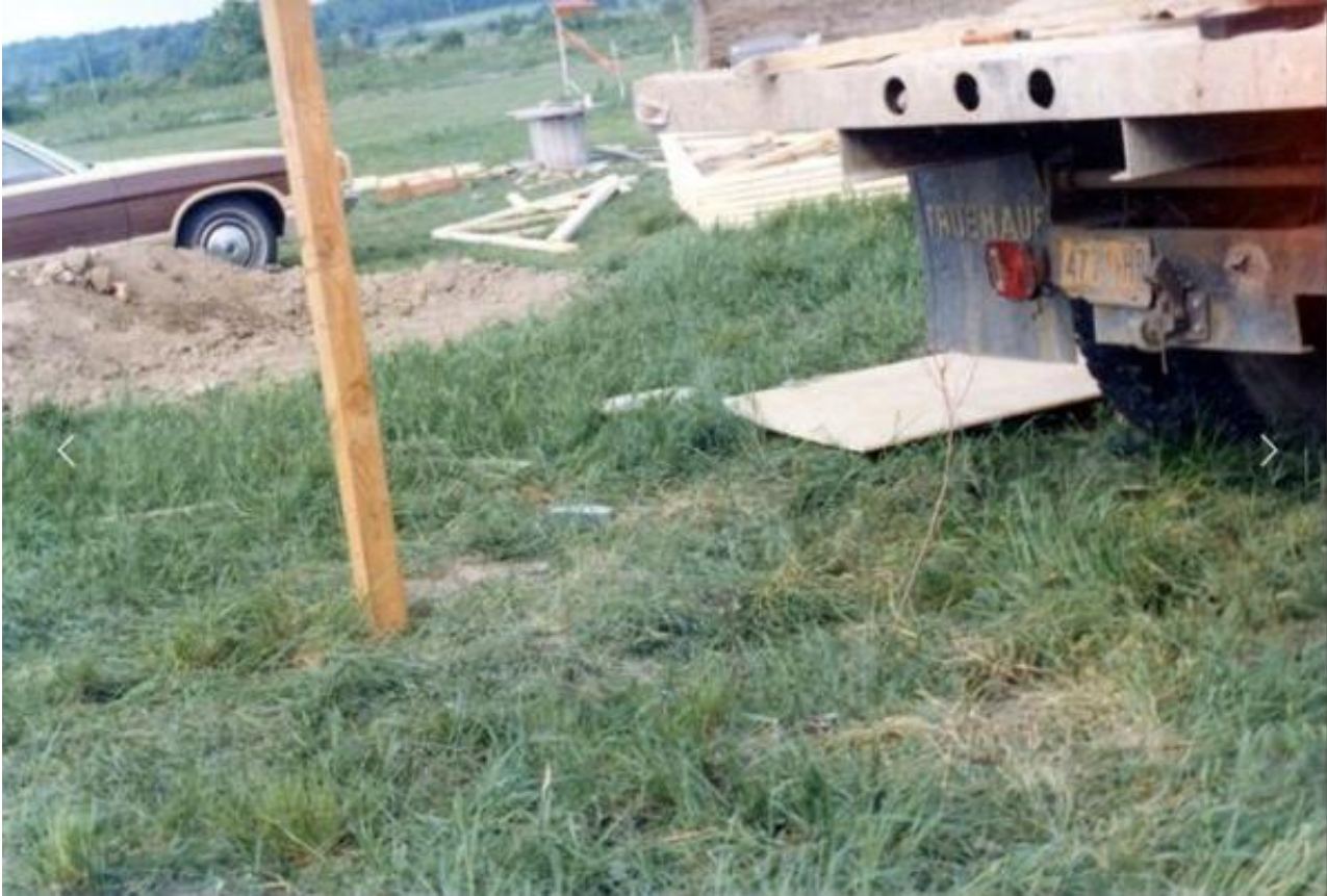
Continuing construction of the pavilion in 1977:
